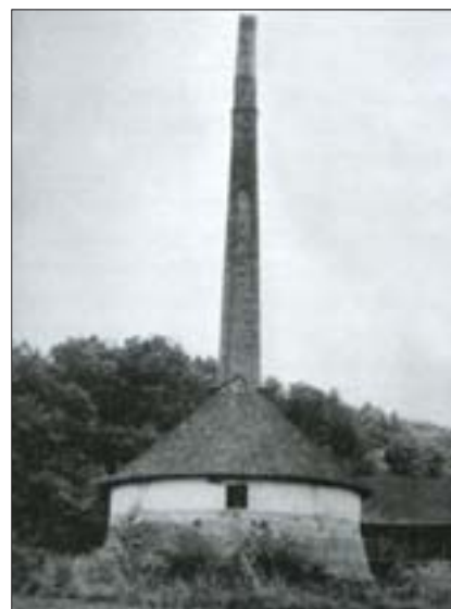
Ringziegelofen in Lutzmannsburg
